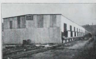
Michigan Central freight house, foot of Third Street, Detroit, built in 12 days.
