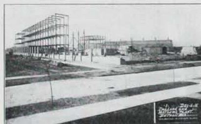
The Ireland & Mathews Manufacturing Co.'s new plant, Detroit.
