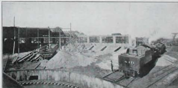
Michigan Central roundhouse and adjoining buildings at Jackson, Mich.
