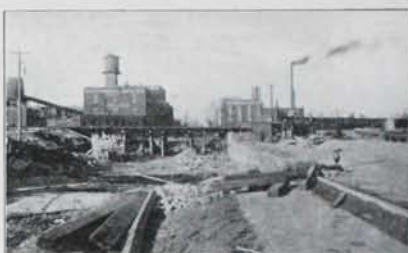
Kirby Avenue East grade separation of the Michigan Central and Grand Trunk tracks, Detroit.
